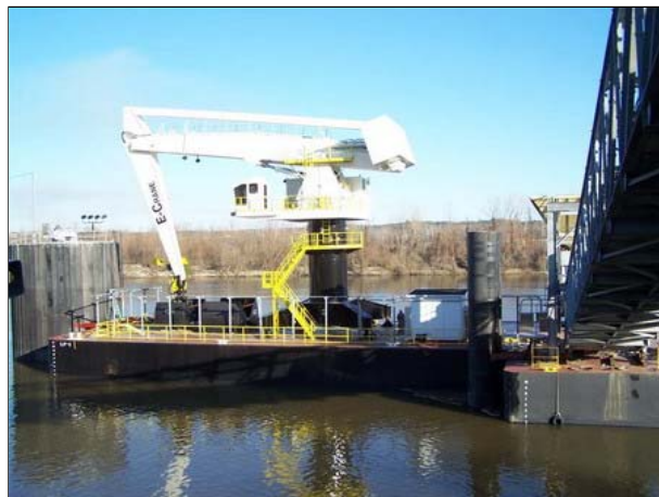
E-Crane floating crane at Lowman Power Station, Alabama
