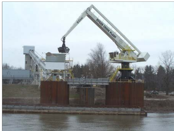
E-Crane - unloader at Kyger Creek
