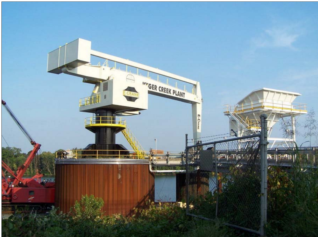
Picture taken by E-Crane International USA during installation
